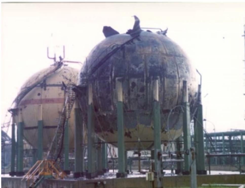
**Photo 1. VCM Plant: heavily damaged VCM storage sphere**
